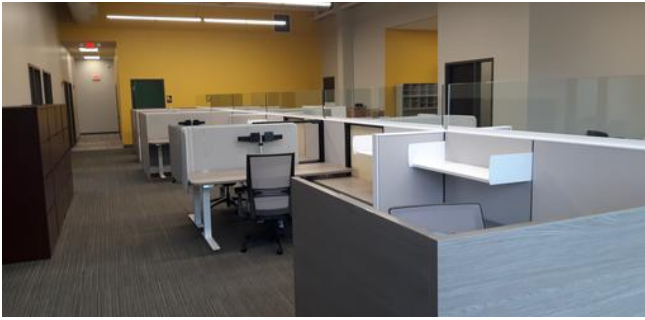
All Systems Installations Apr 21, 2021 3:57 PM
