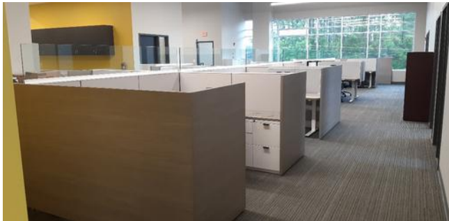
20210420_143710_resized All Systems Installations Apr 22, 2021 12:57 PM
