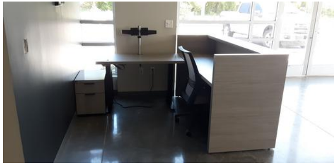
All Systems Installations Apr 21, 2021 3:59 PM
