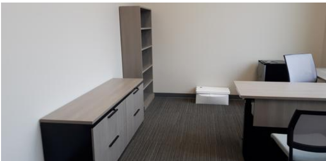
All Systems Installations Apr 21, 2021 3:57 PM
